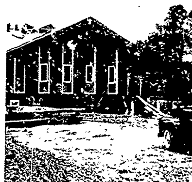
One of the buildings of a new State boys' camp under construction just west of Walsenburg. The facility will be an important addition to the area's economy.
